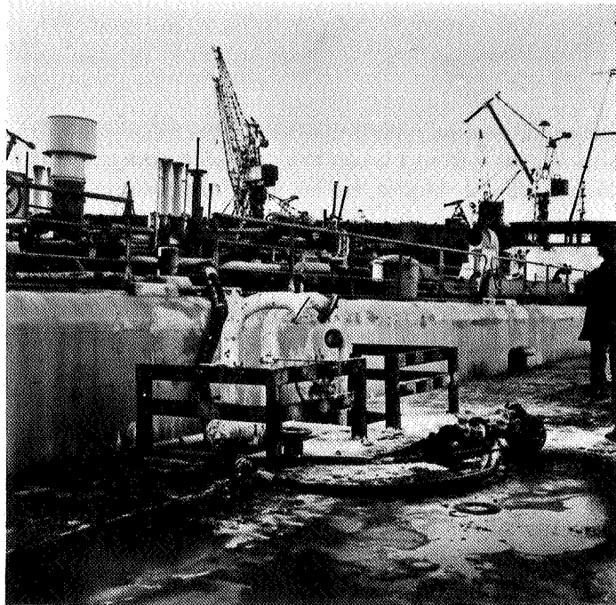
Figure 5. Condition of connections after the accident.
